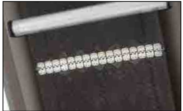
Fig 52 - Conveyor belt seam under tube
