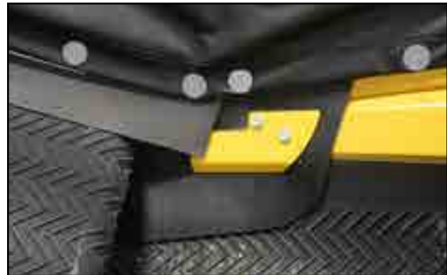
Fig 68 - Fasten flashing clamp
