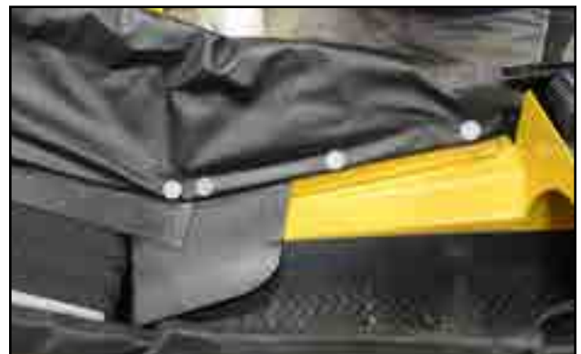
Fig 65 - Transition corner flashing in place
