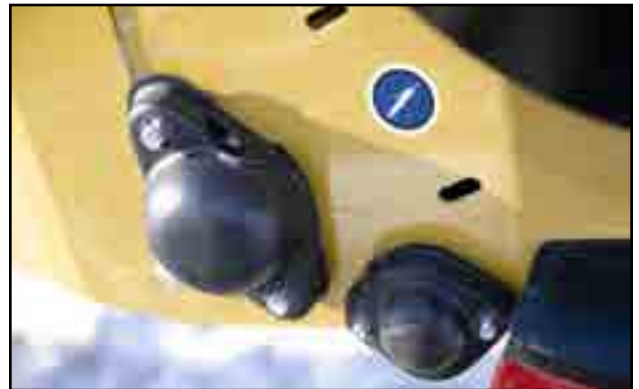
Fig 36 - Discharge roller bearings
